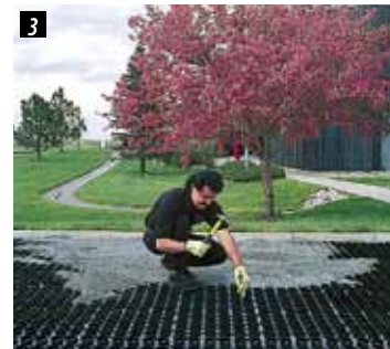
3 Secure mats with anchors provided (size and type may vary).
