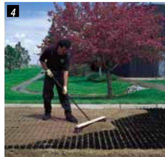
4 Fill rings with clean sharp concrete sand.
