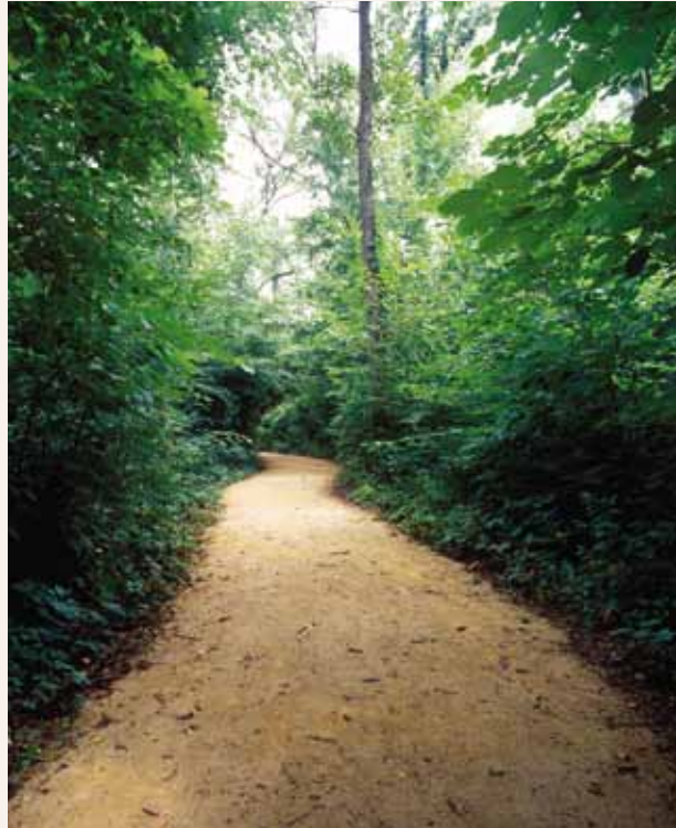
Oakdale Nature Preserve, Freeport, Illinois—Gravelpave 2 reduces erosion and rutting in this ADA accessible trail.
