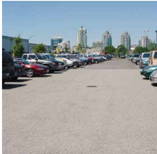
Vancouver City Works Yard, Vancouver, British Columbia—main staff parking lot, done in Gravelpave 2 .
