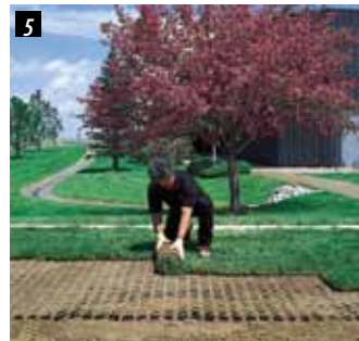
5 Hydroseed or lay sod.
