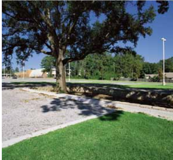
The University of South Alabama, Mobile used Gravelpave 2 in parking aisles and Grasspave 2 in the spaces.
