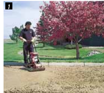
1 Place and compact sand and gravel road base.
