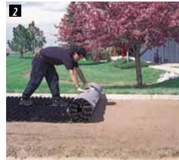
2 Roll out Gravelpave 2 , aligning the snap fit fasteners.
