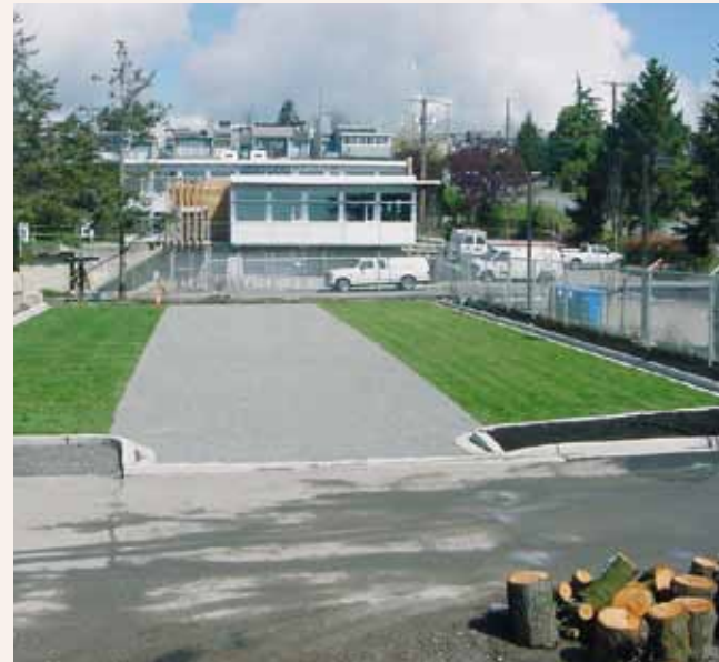
City of White Rock Operations, White Rock, British Columbia—Gravelpave 2 is used in the main drive aisle of the works yard and Grasspave 2 is used for the parking bays.
