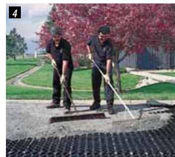
4 Fill rings with clean gravel.
