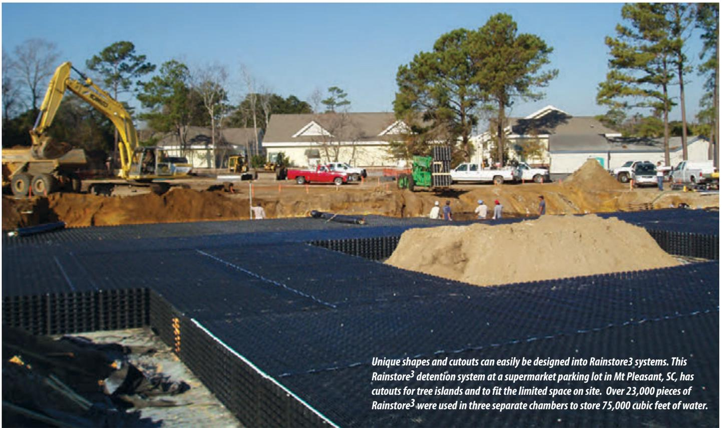
*Unique shapes and cutouts can easily be designed into Rainstore<sup>3</sup> systems. This Rainstore<sup>3</sup> detention system at a supermarket parking lot in Mt Pleasant, SC, has cutouts for tree islands and to fit the limited space on site. Over 23,000 pieces of Rainstore<sup>3</sup> were used in three separate chambers to store 75,000 cubic feet of water.*
