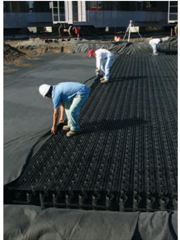
*Above: Workers cover Rainstore<sup>3</sup> units with geogrid and geotextile fabric at Adams Street Station in Jacksonville, FL. Two separate Rainstore<sup>3</sup> detention chambers were designed at only 2 units high (20 cm) to account for the high water table.*
