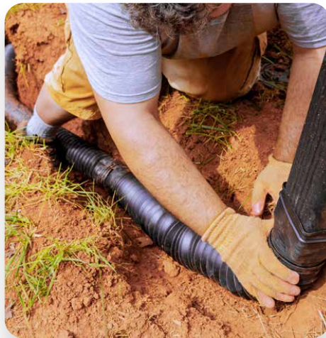
Downspout Catch Basins
