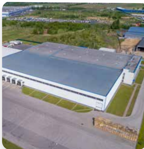
Ramps, Docks & Loading Areas
