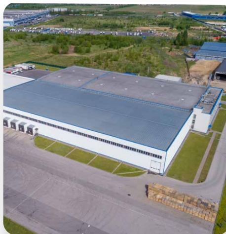
Ramps, Docks & Loading Areas
