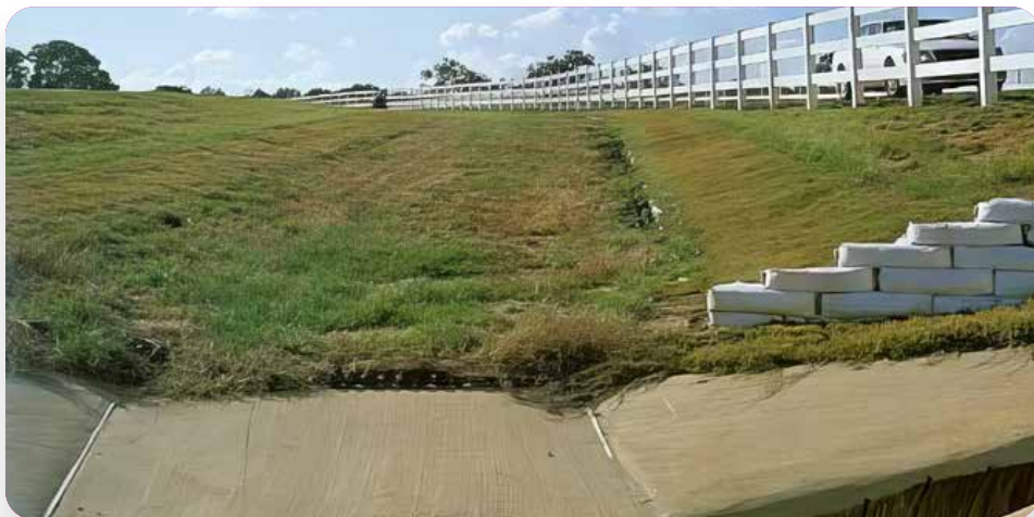
Stormwater Infiltration Trenches
